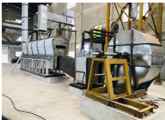
Erection of Table Salt Plant
